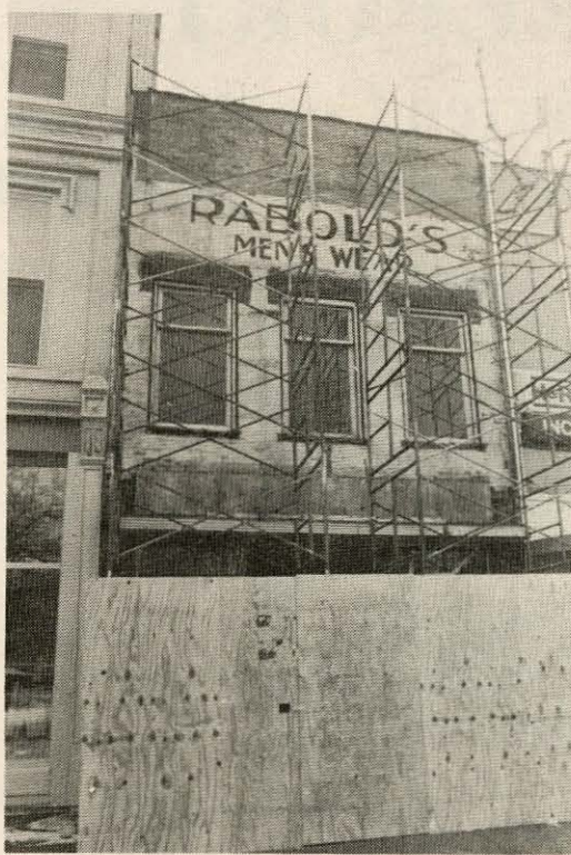
BARCLAY BUILDING 426 EAST MAIN STREET
