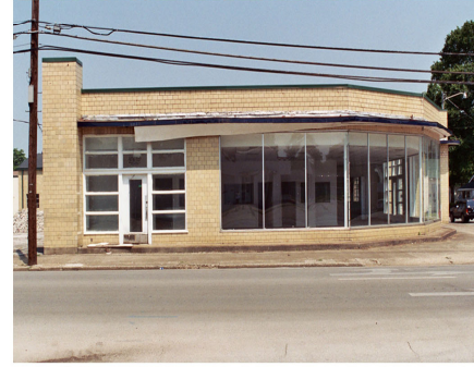
SHOWROOM EXTERIOR WALL
