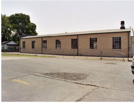
WAREHOUSE EXTERIOR WALL
