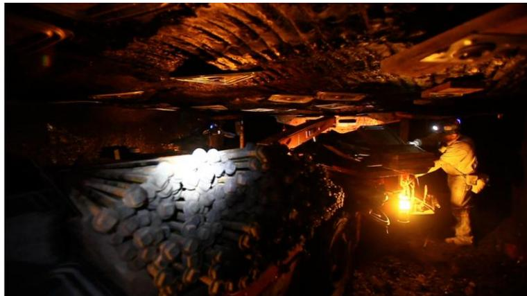
**Figure 6.2** Kevin Brown, of Boxville, Ky., pins the ceiling of a recently mined area.
