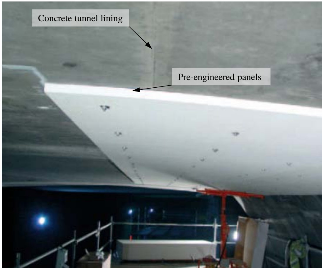
Figure 15. Installation of Promat®-T panels in the Toulon Tunnel, France (Promat International 2005).
