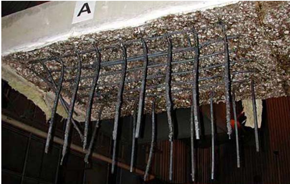
Figure 2. Severe spalling of reinforced concrete member after exposure to elevated temperatures (Boström and Larsen 2006).
