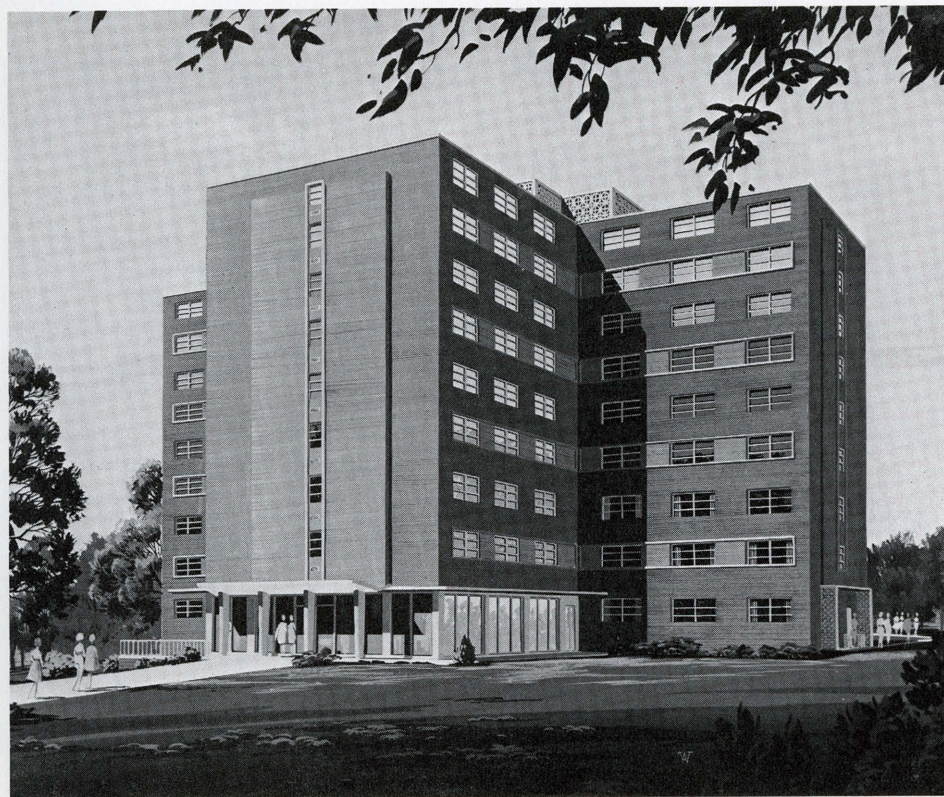
New Dormitory for Women (now under construction)
