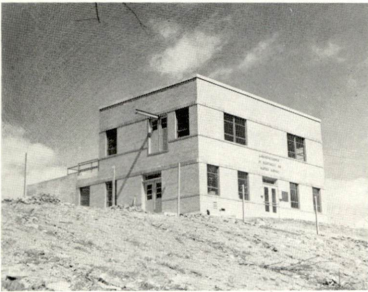
City of Lawrenceburg Water Plant
