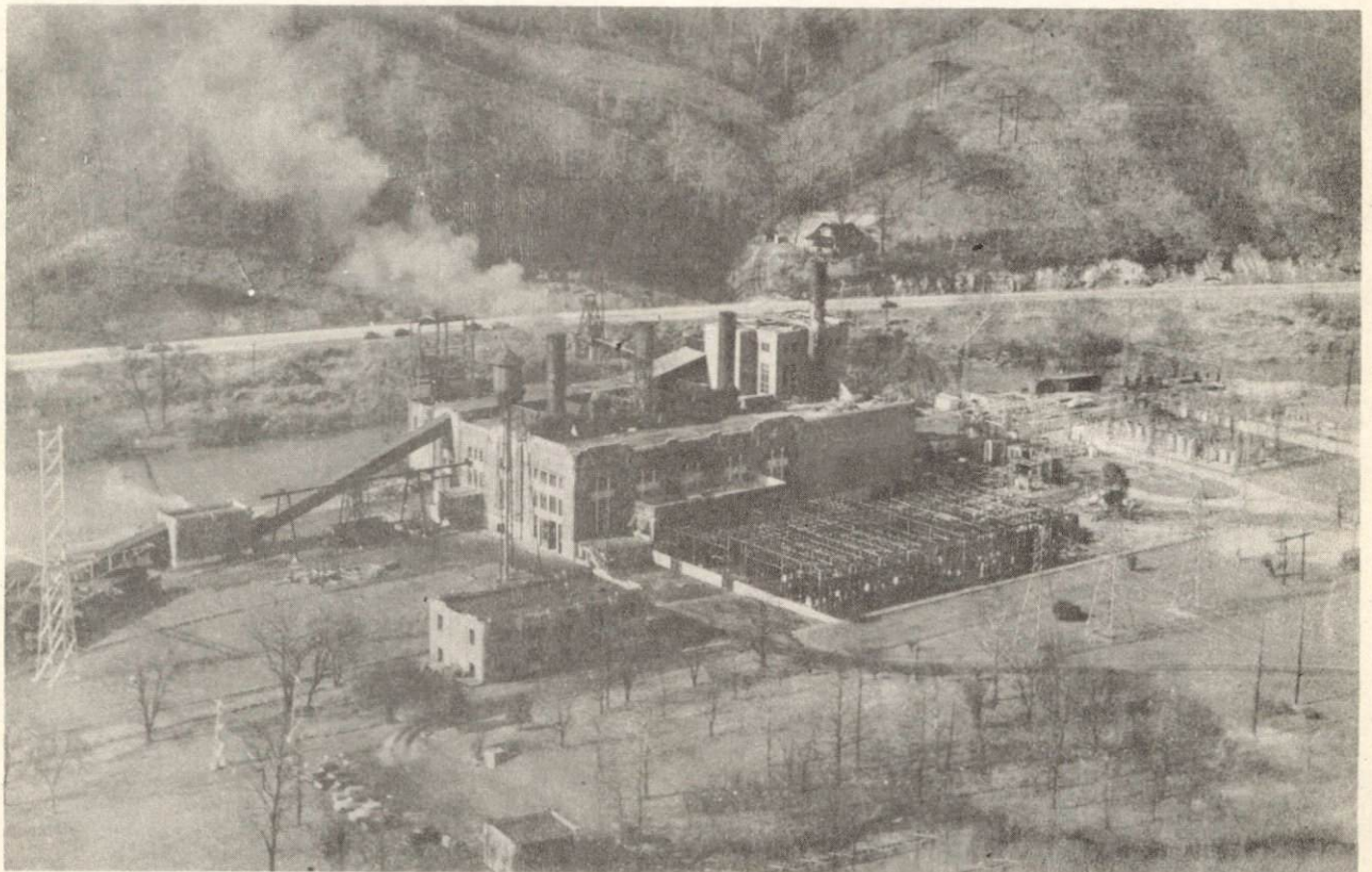
KENTUCKY UTILITIES STEAM GENERATION PLANT
