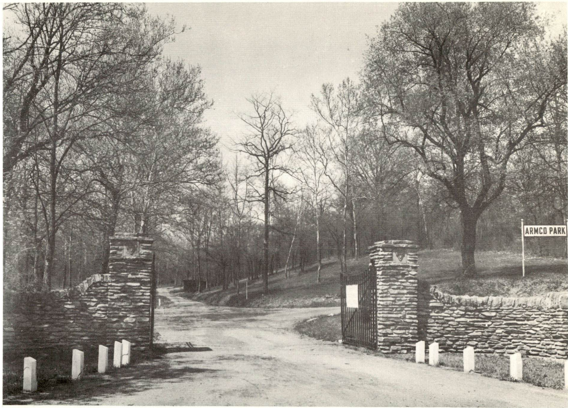
Entrance to Armco Park, Ashland, Kentucky
