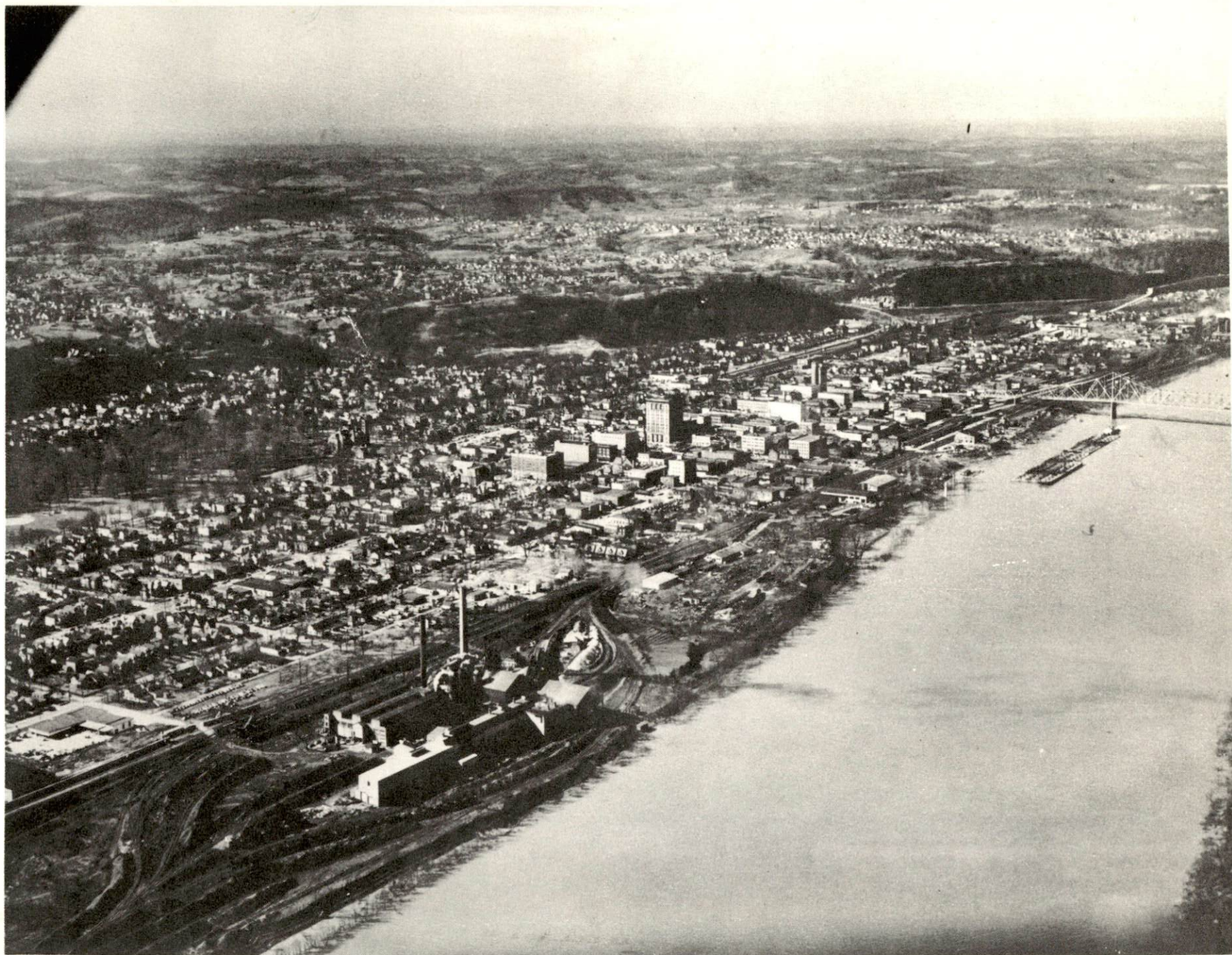
Aerial View of Ashland, Kentucky
