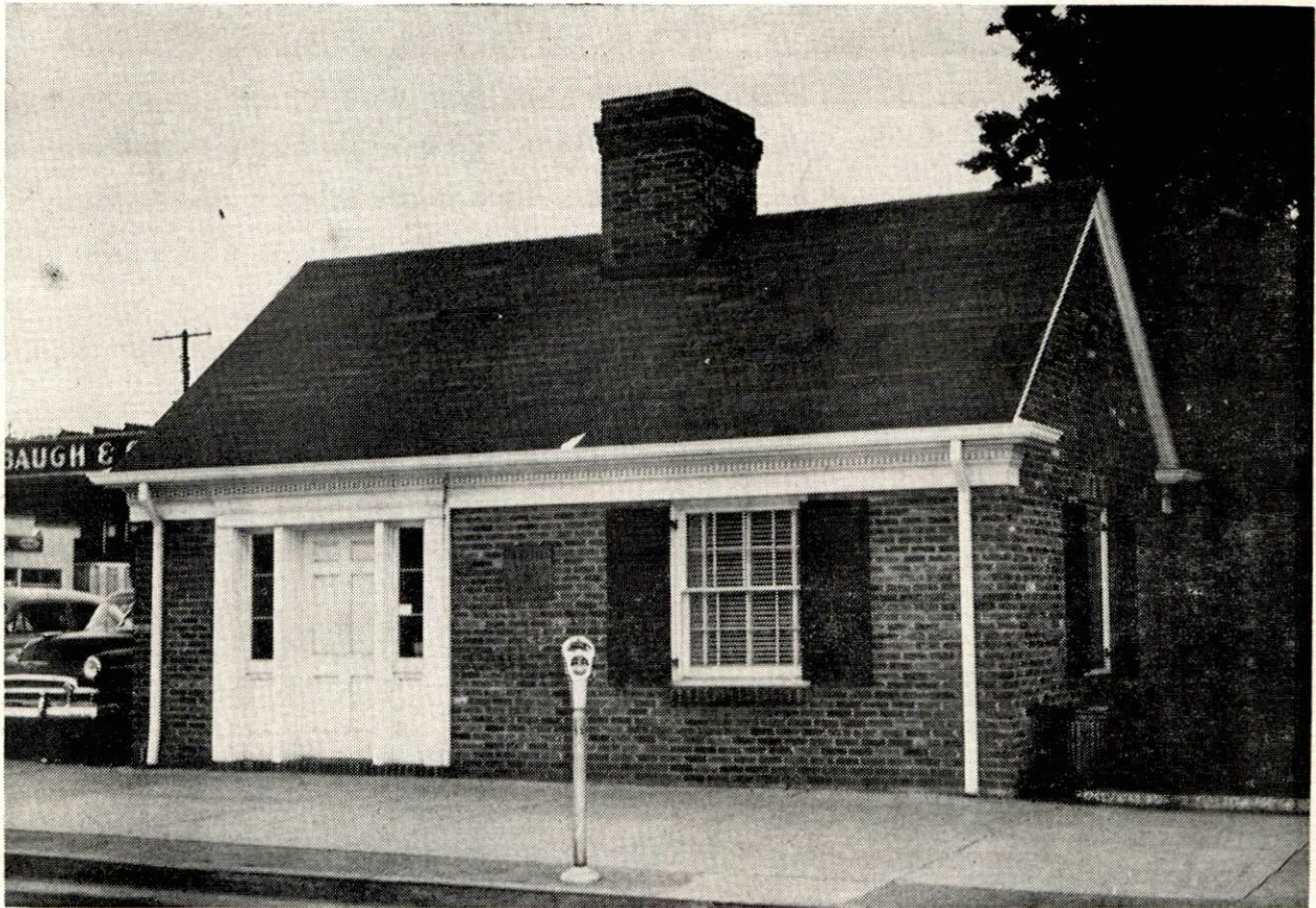
CHAMBER OF COMMERCE OFFICE
