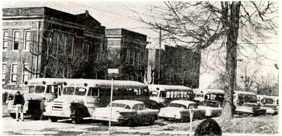
Morgantown Elementary School
