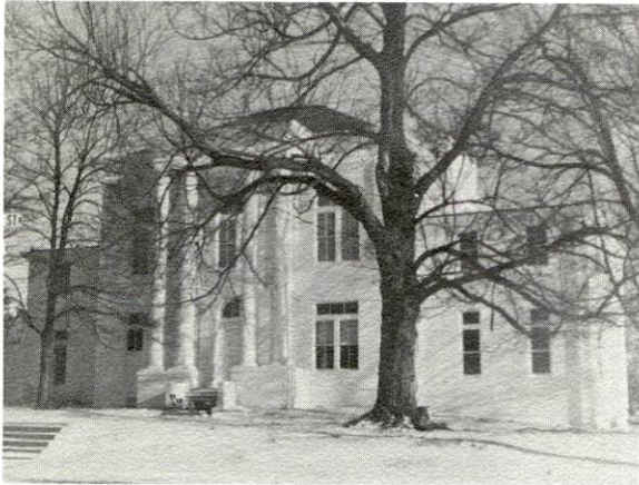
Carlisle County Court House
