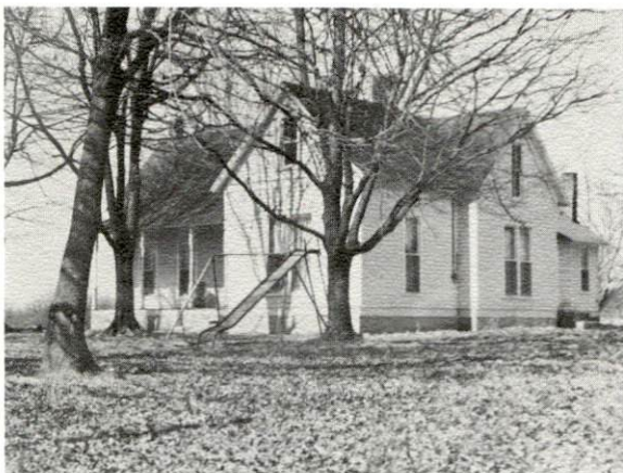
Community Center and Kindergarten
