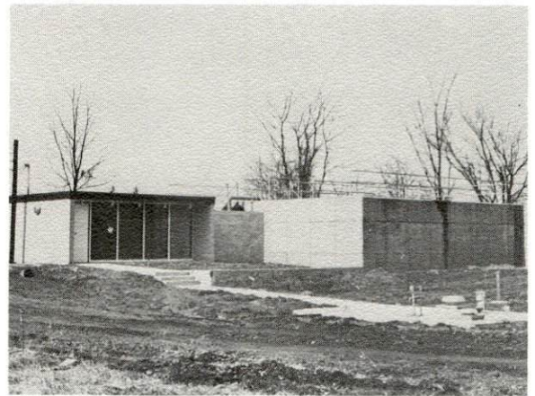
Sewage Disposal Plant
