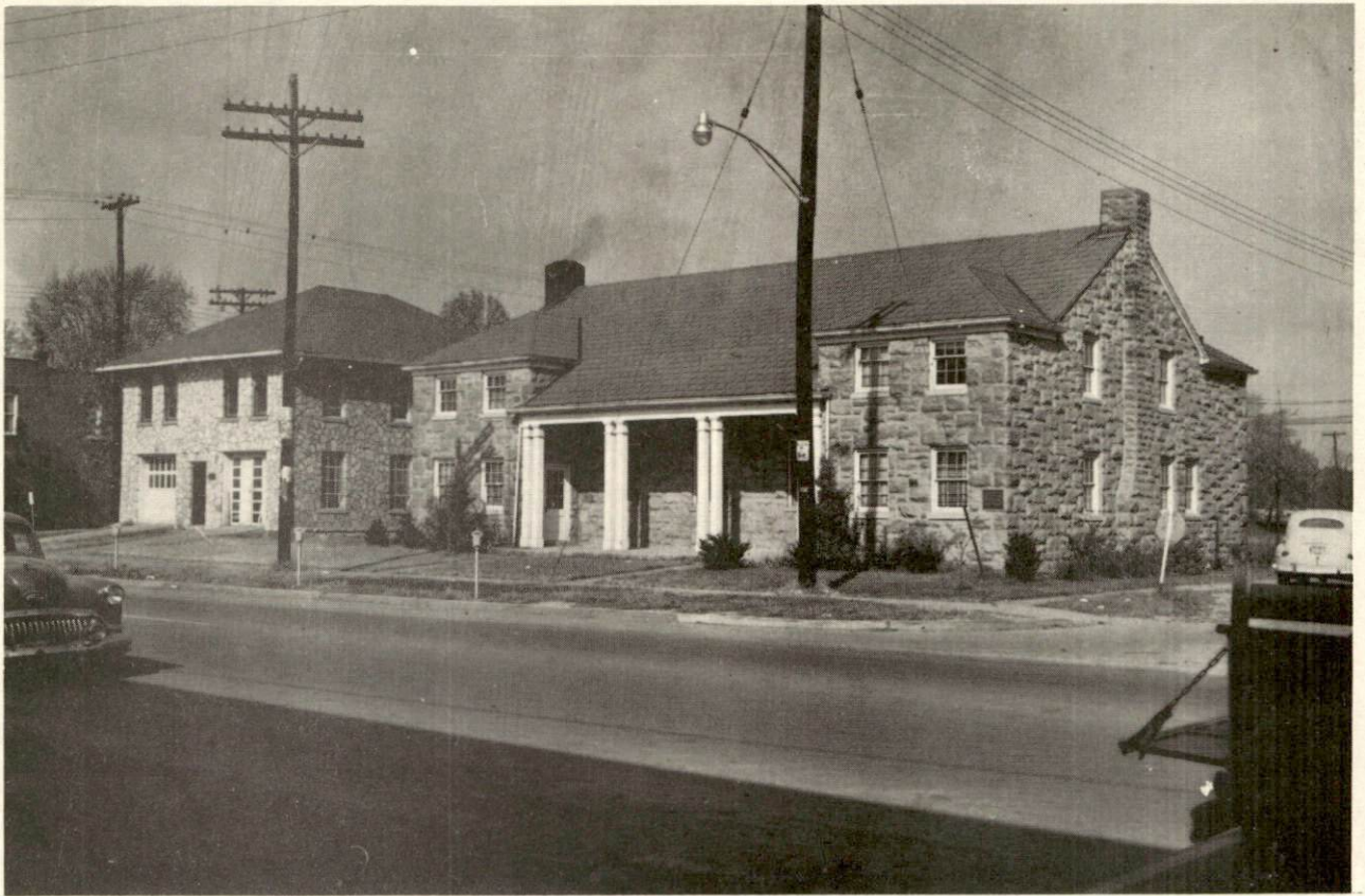
GRAYSON COMMUNITY BUILDING
