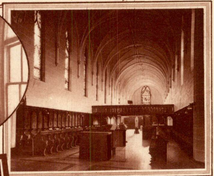
Nave of Church.
