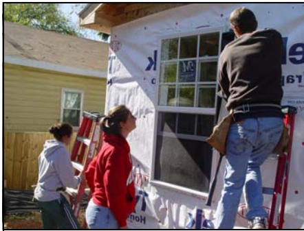
Featured above: WKU Habitat for Humanity Chapter working on the Centennial Build.
