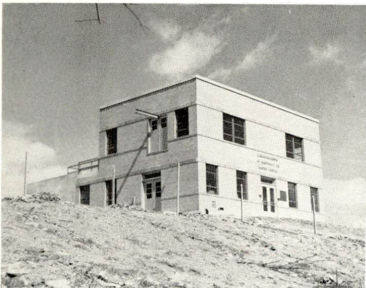
Municipal Water Plant
