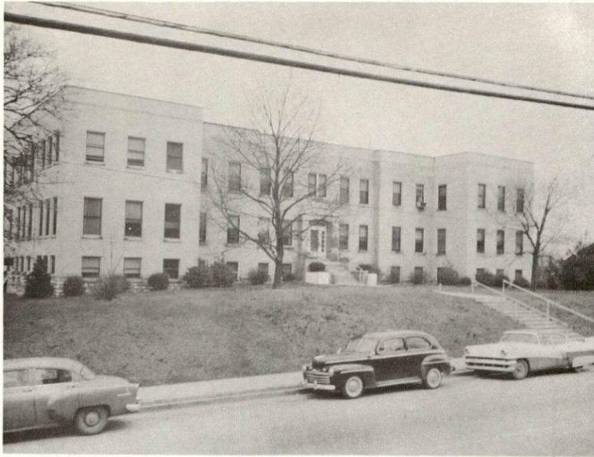
CLARK COUNTY HOSPITAL
