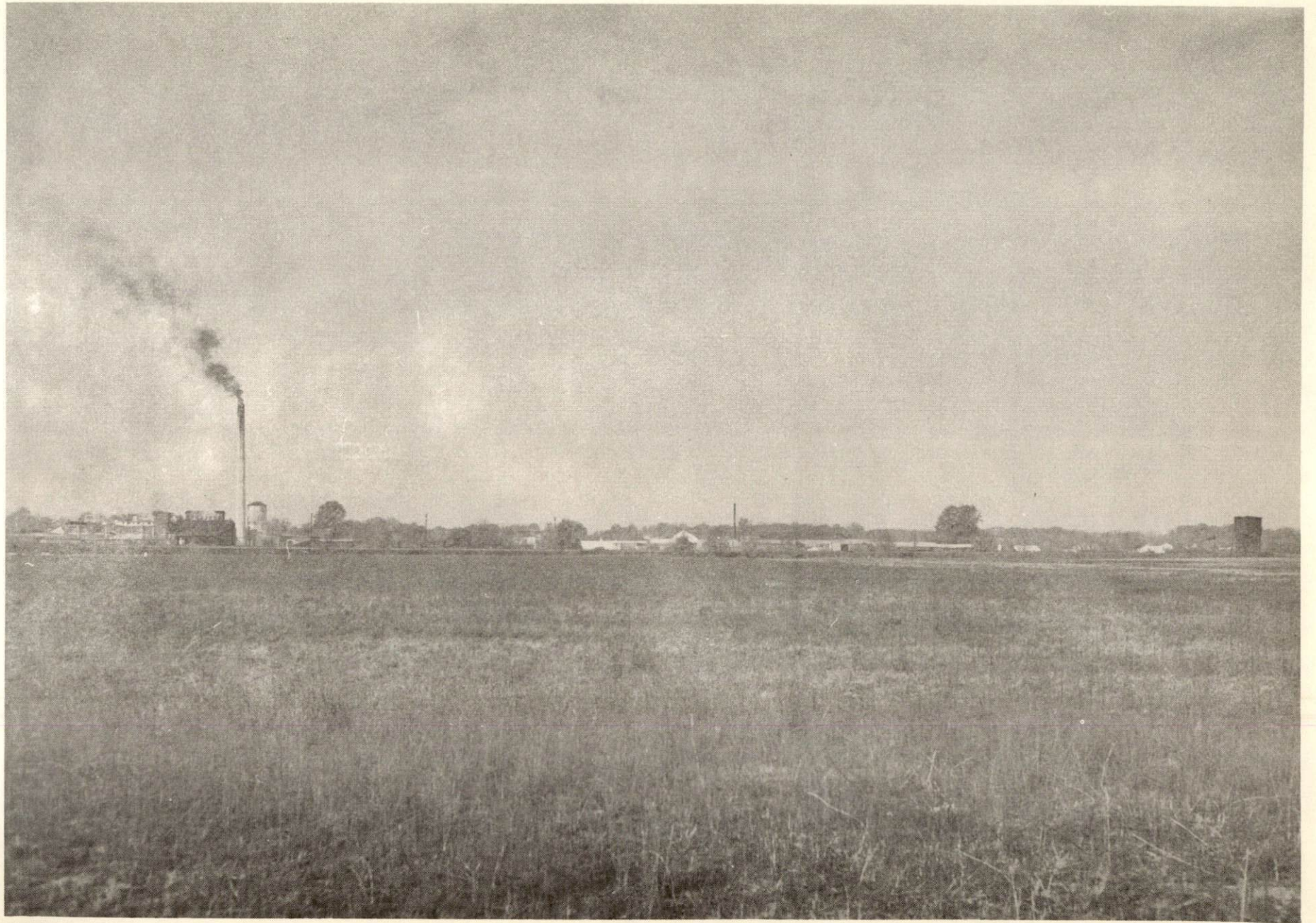
INDUSTRIAL SITE NO. 3
