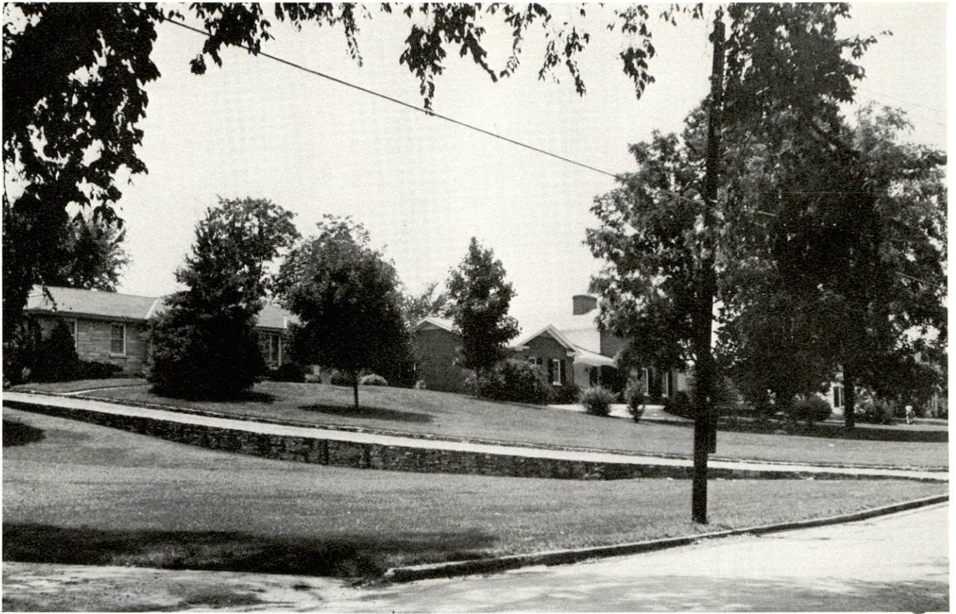
Greensburg Residential Area
