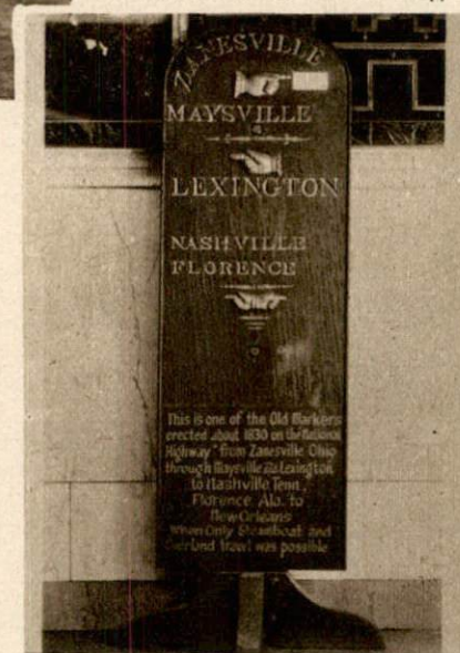
One of the old iron markers erected about 1830 at every mile along the Maysville Pike, which is the oldest macadam highway in the state; now U. S. Highway No. 68.
