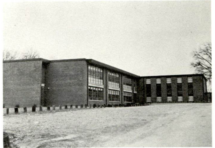
ALLEN COUNTY ELEMENTARY SCHOOL
