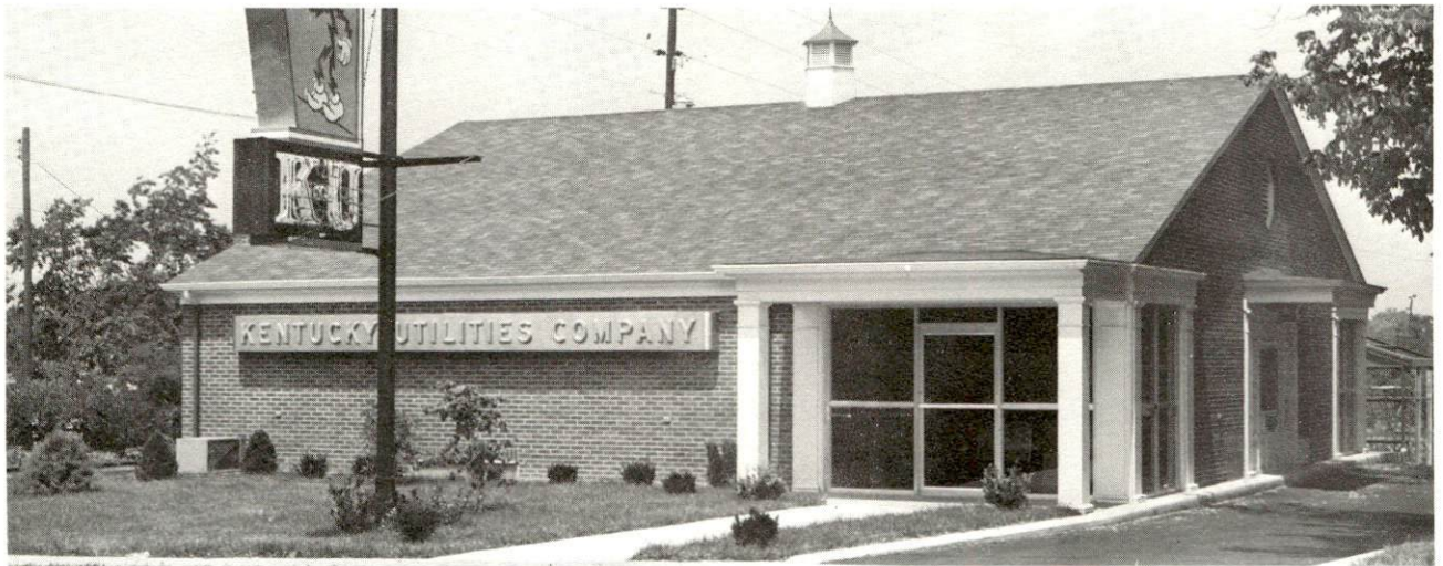
KENTUCKY UTILITIES COMPANY OFFICE
