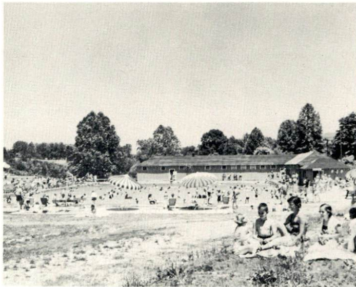
ASHLAND CITY SWIMMING POOL
