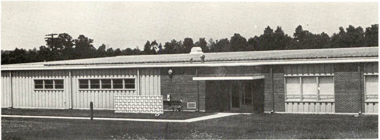
EDMONTON MANUFACTURING COMPANY
