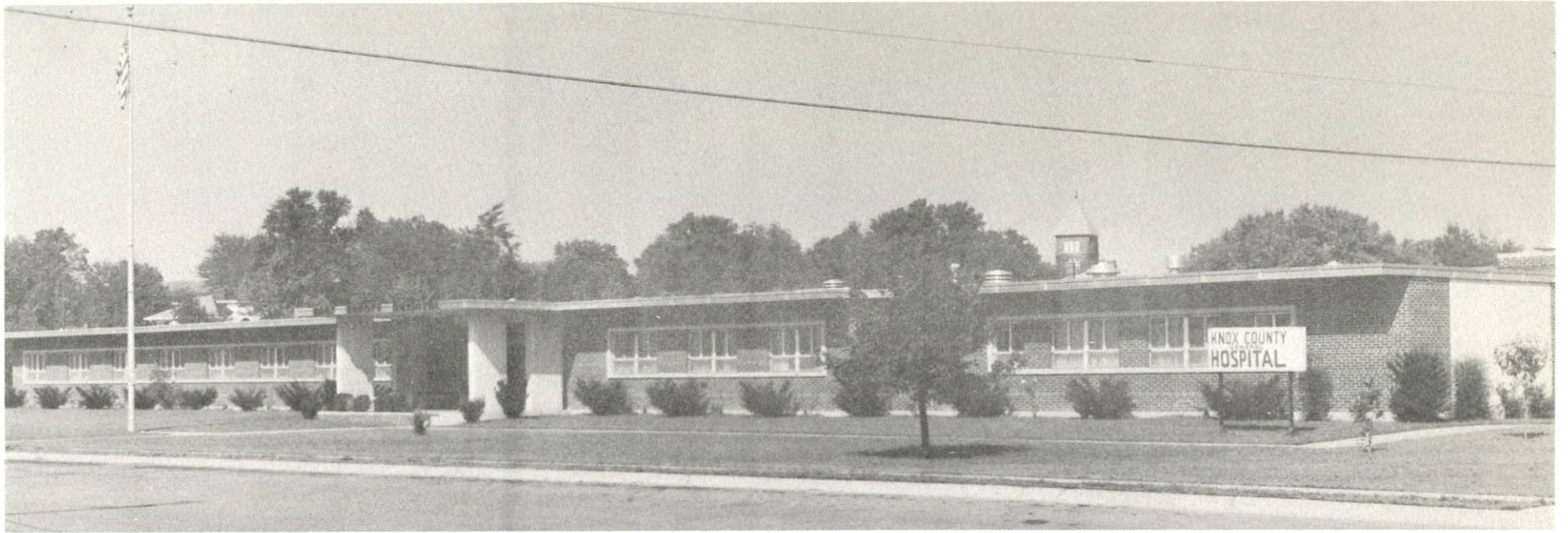
KNOX COUNTY HOSPITAL
