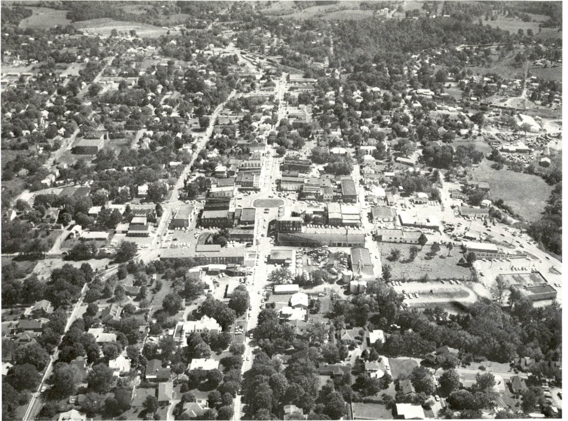
AERIAL VIEW OF SCOTTSVILLE, KENTUCKY
