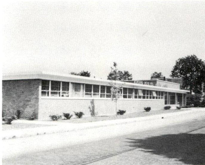
ASHLAND - BOYD COUNTY HEALTH CENTER
