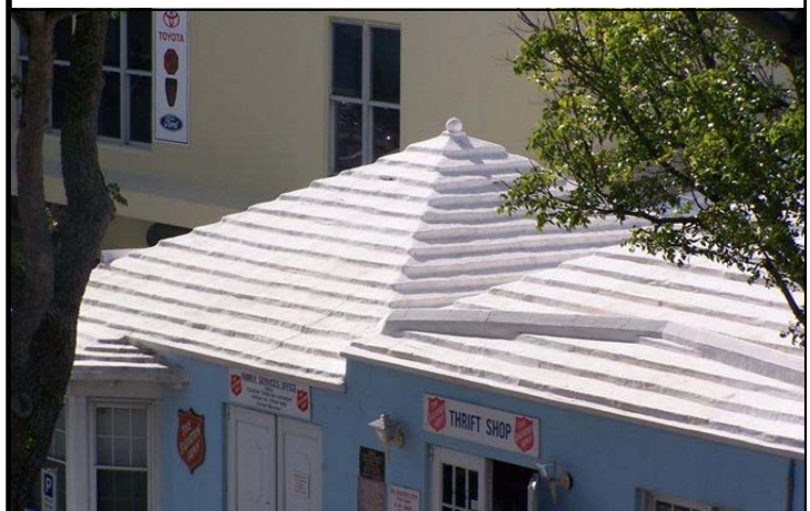
Characteristic white, lime stucco roofs are designed to catch rainwater and direct it into a basement cistern for personal use.
