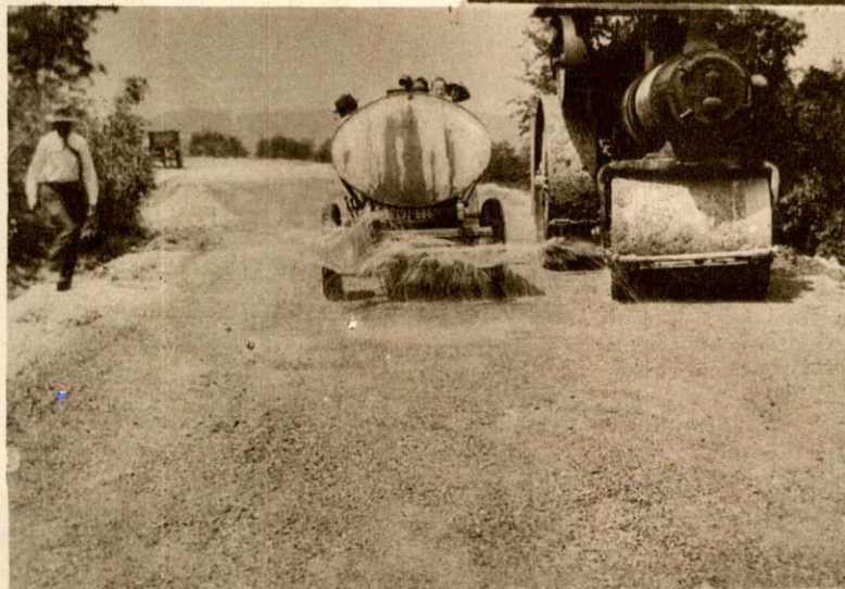
Making waterbound macadam between Owenton and Carrollton.
