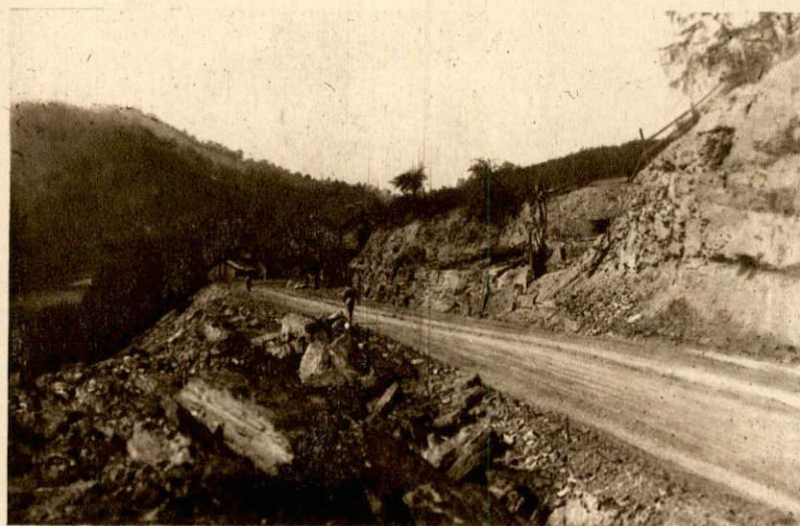
Finished stretch near Jackson in Breathitt county.
