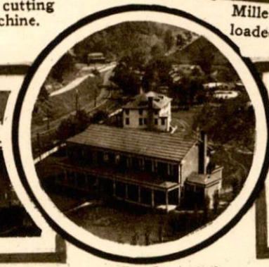
Recreation building, Van Lear, Ky.
