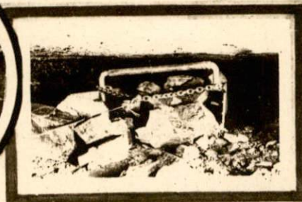
Coal being brought to entry by scoop.
