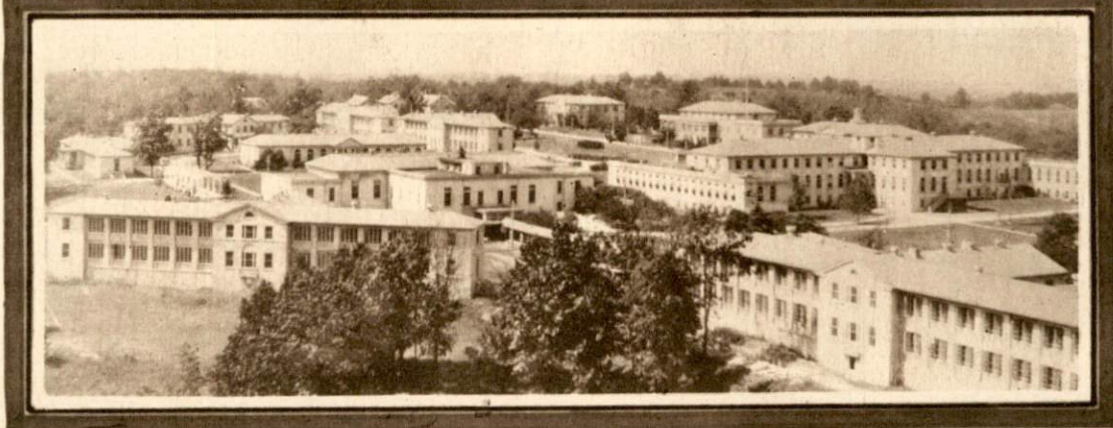
General view of a section of the hospital buildings.
