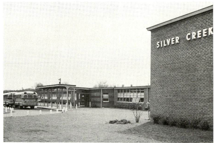
SILVER CREEK ELEMENTARY SCHOOL
