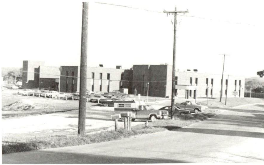
Morgan County Appalachian Regional Hospital
