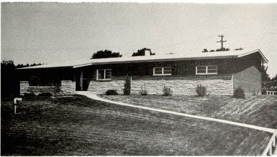
The New Duo-County Telephone Cooperative Corp. Office Building located in Jamestown.
