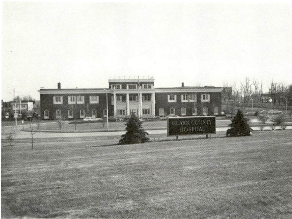
CLARK COUNTY HOSPITAL
