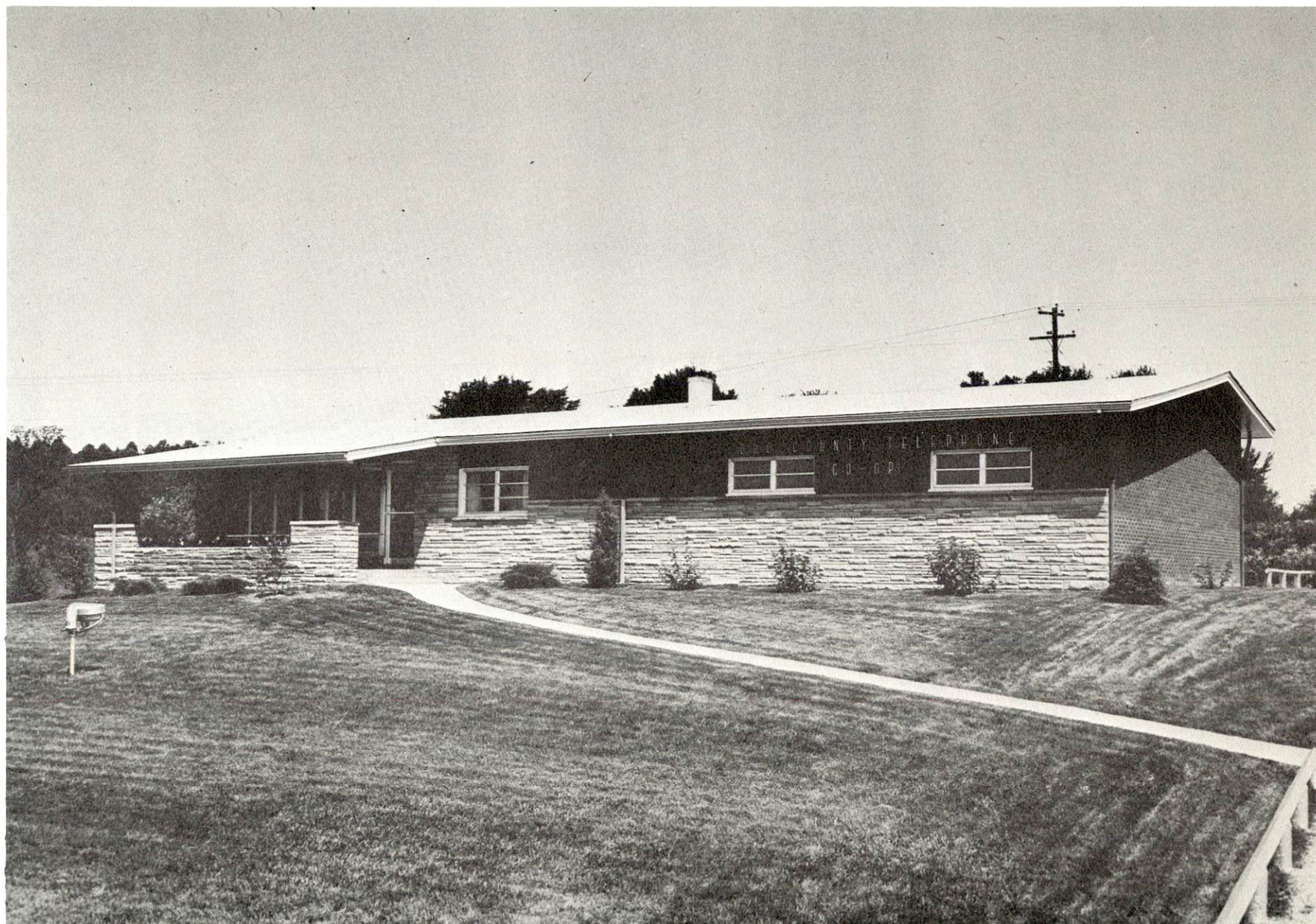
New Duo County Telephone Cooperative Corp. office building located in Jamestown
