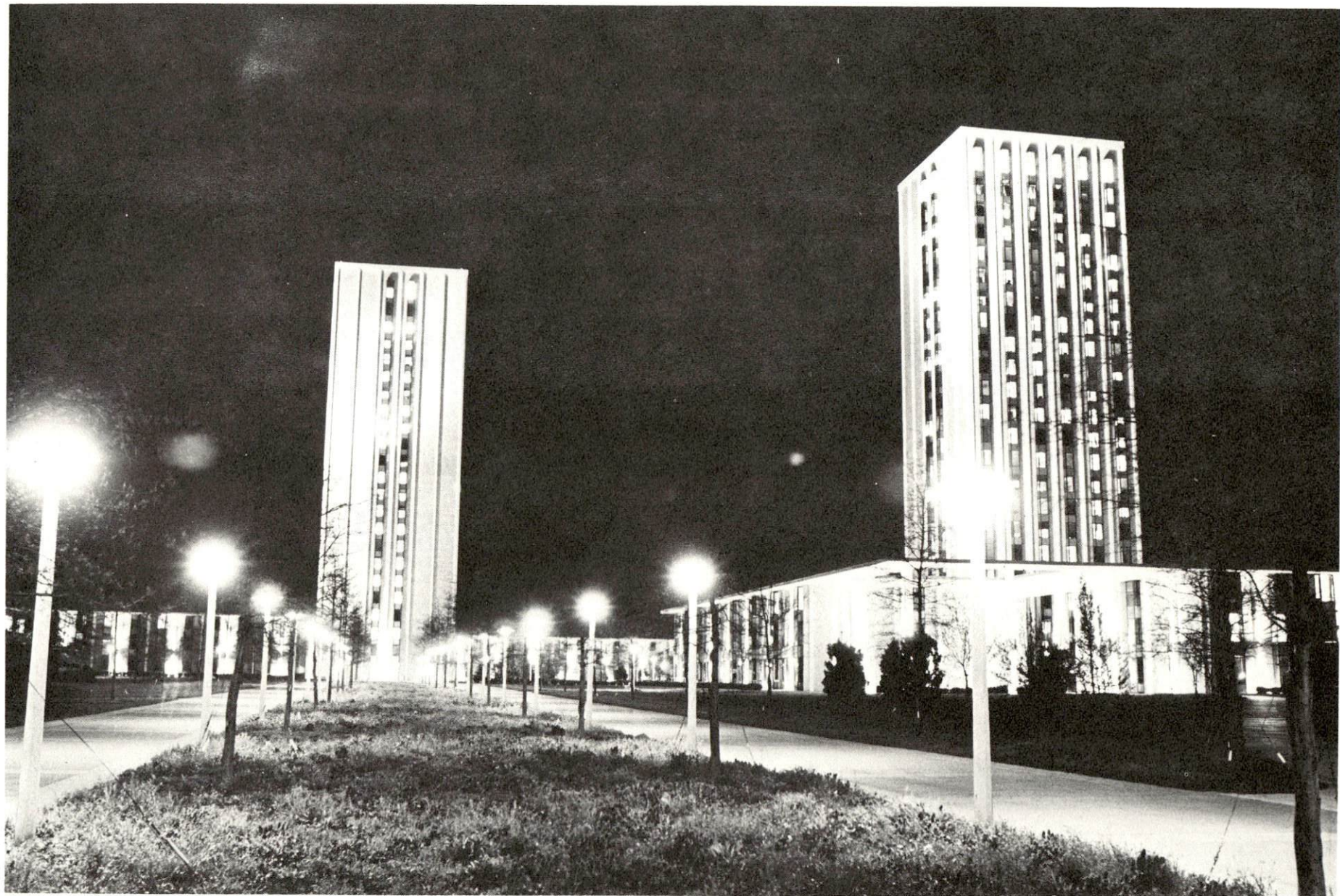
BLANDING-KIRWAN DORMITORY COMPLEX UNIVERSITY OF KENTUCKY
