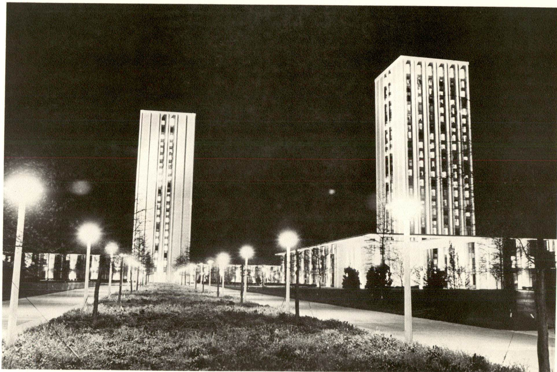
BLANDING-KIRWAN DORMITORY COMPLEX UNIVERSITY OF KENTUCKY
