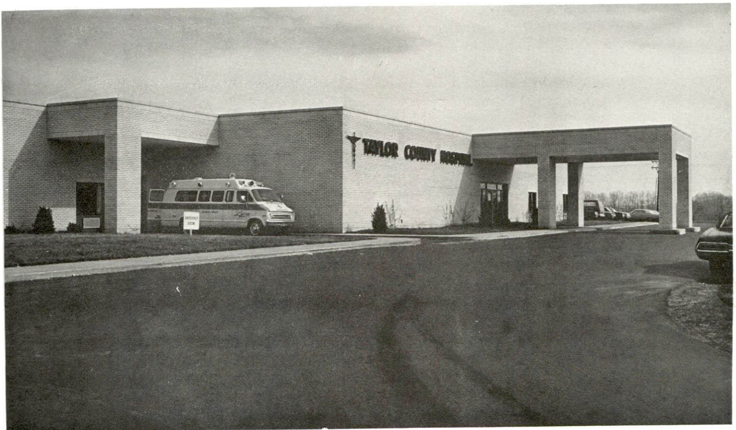
TAYLOR COUNTY HOSPITAL
