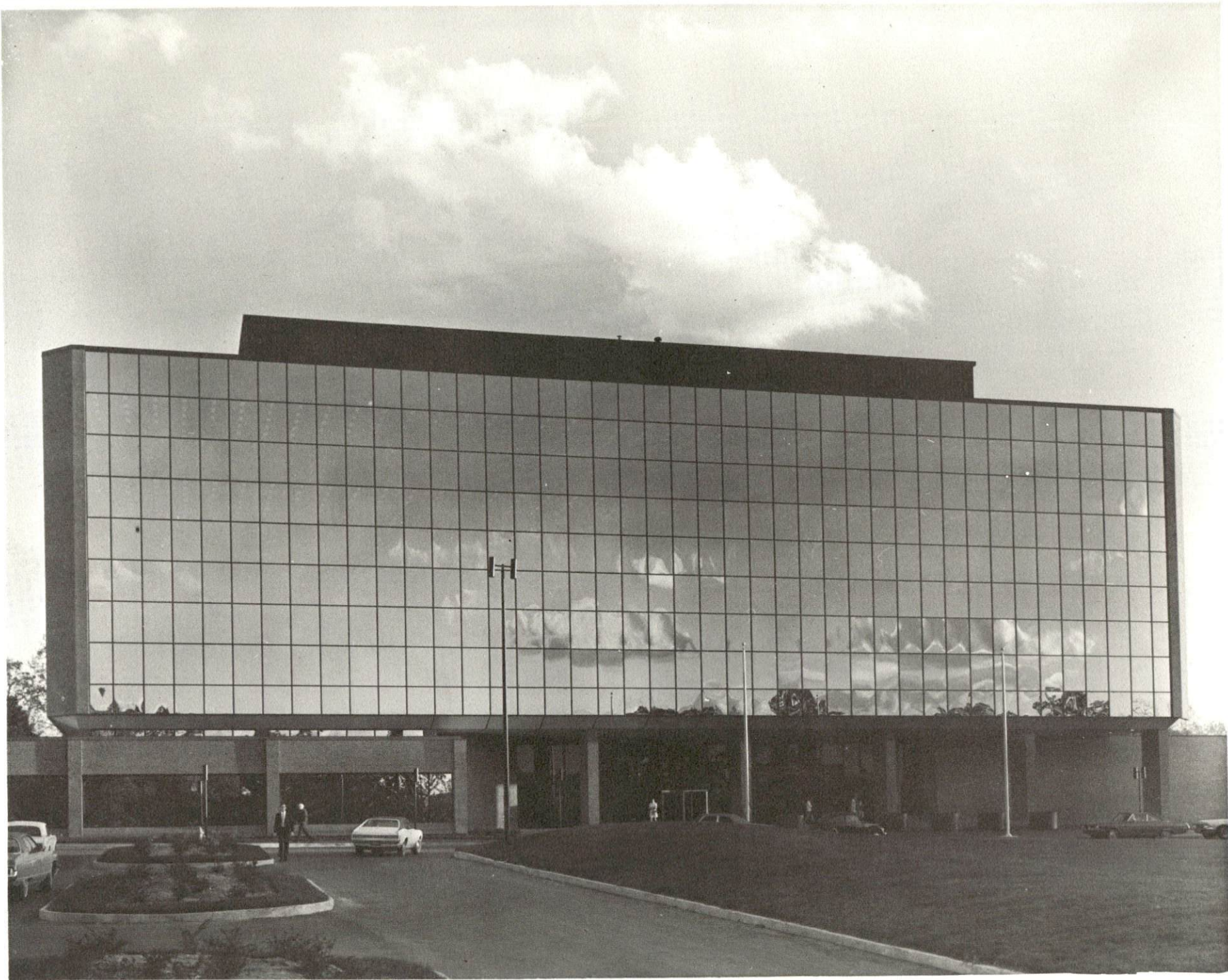
ASHLAND OIL'S NEW EXECUTIVE HEADQUARTERS.
