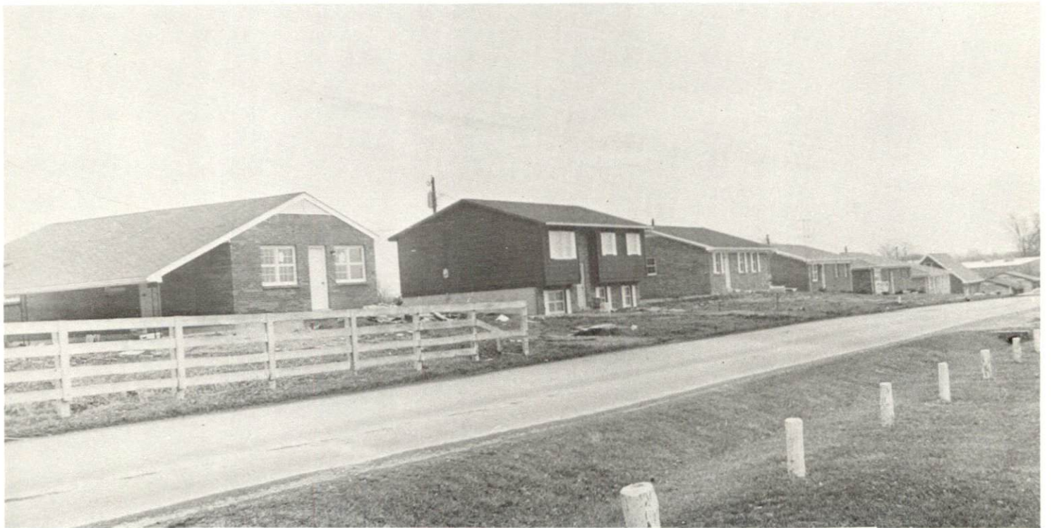
NEW RESIDENTIAL CONSTRUCTION
