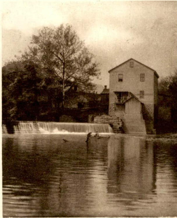
Flour mill and dam at Robinson, near Cynthiana.
