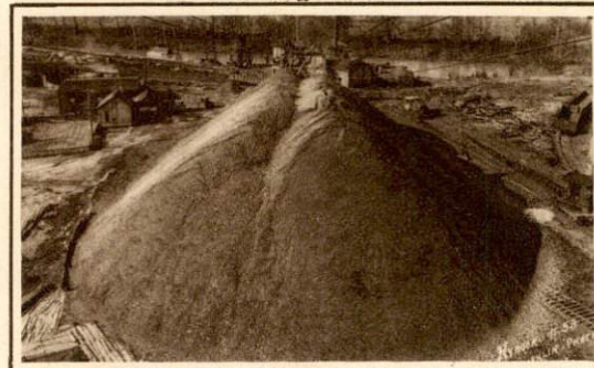
Stock pile of Kentucky rock asphalt. 200,000 tons in storage to insure prompt deliveries during road building season.
