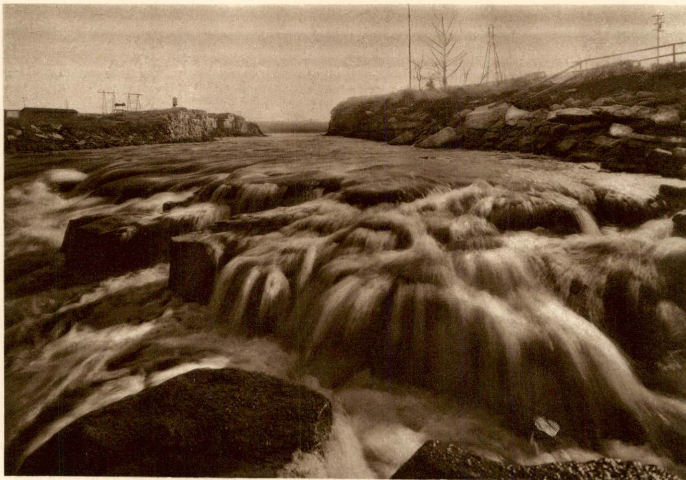
Spillway, Dix Dam. The lake above dam is a fisherman's paradise.
