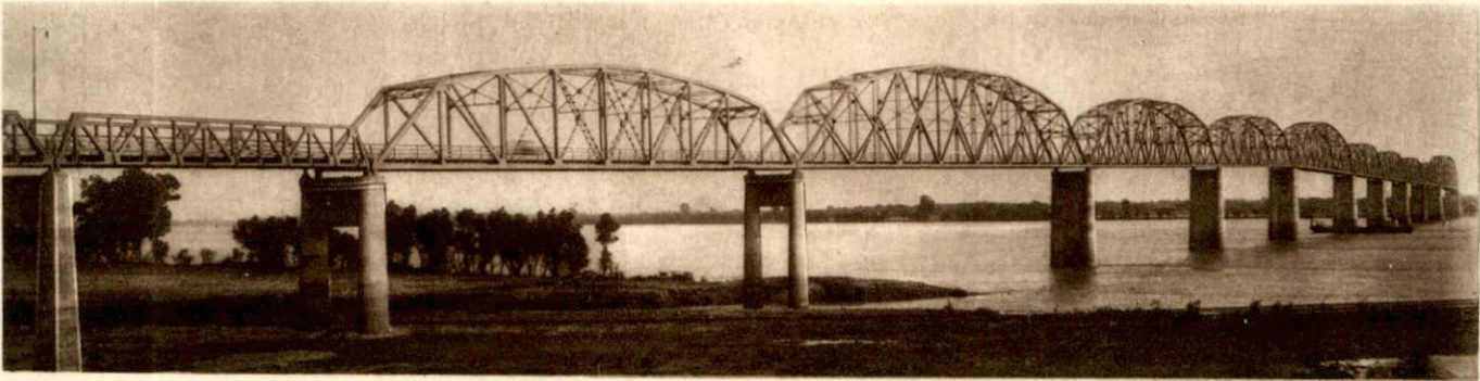
New Paducah-Ohio River bridge on U. S. No. 45.
