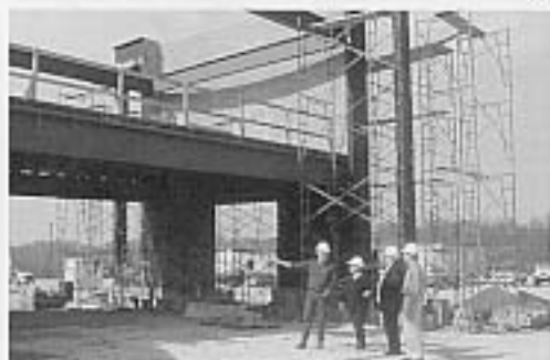
The new Glasgow Library under construction
