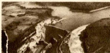
Dix Dam, Harrodsburg, Ky. Largest rock-filled dam in the world.
