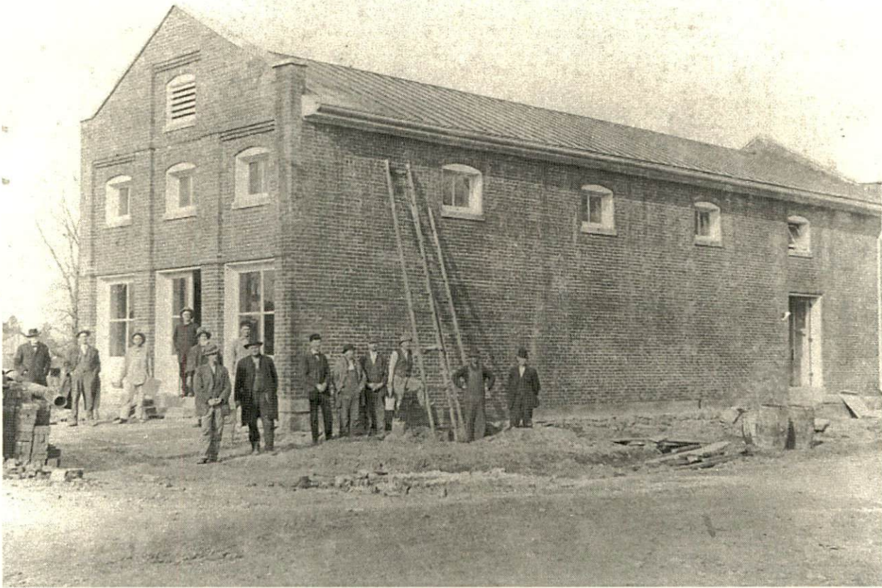
1896 Shaker Store & Post Office (Under Construction)
