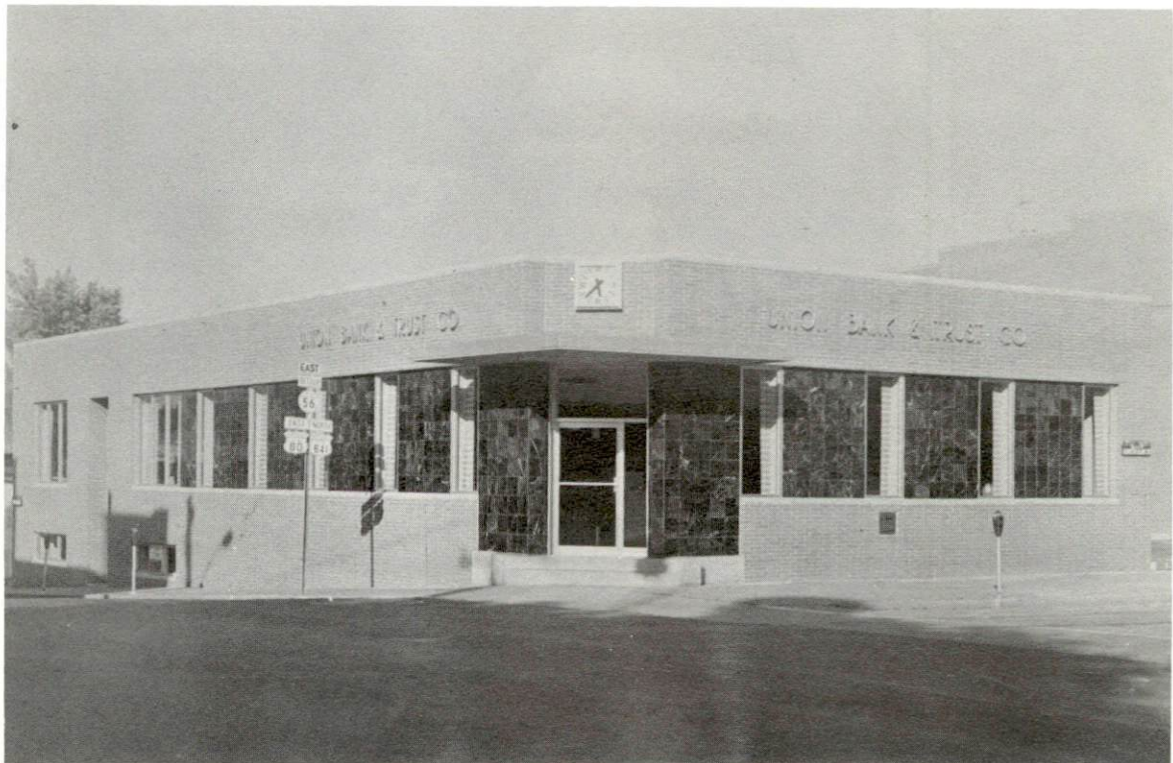
UNION BANK AND TRUST COMPANY - COMPLETELY RENOVATED INSIDE AND OUTSIDE
