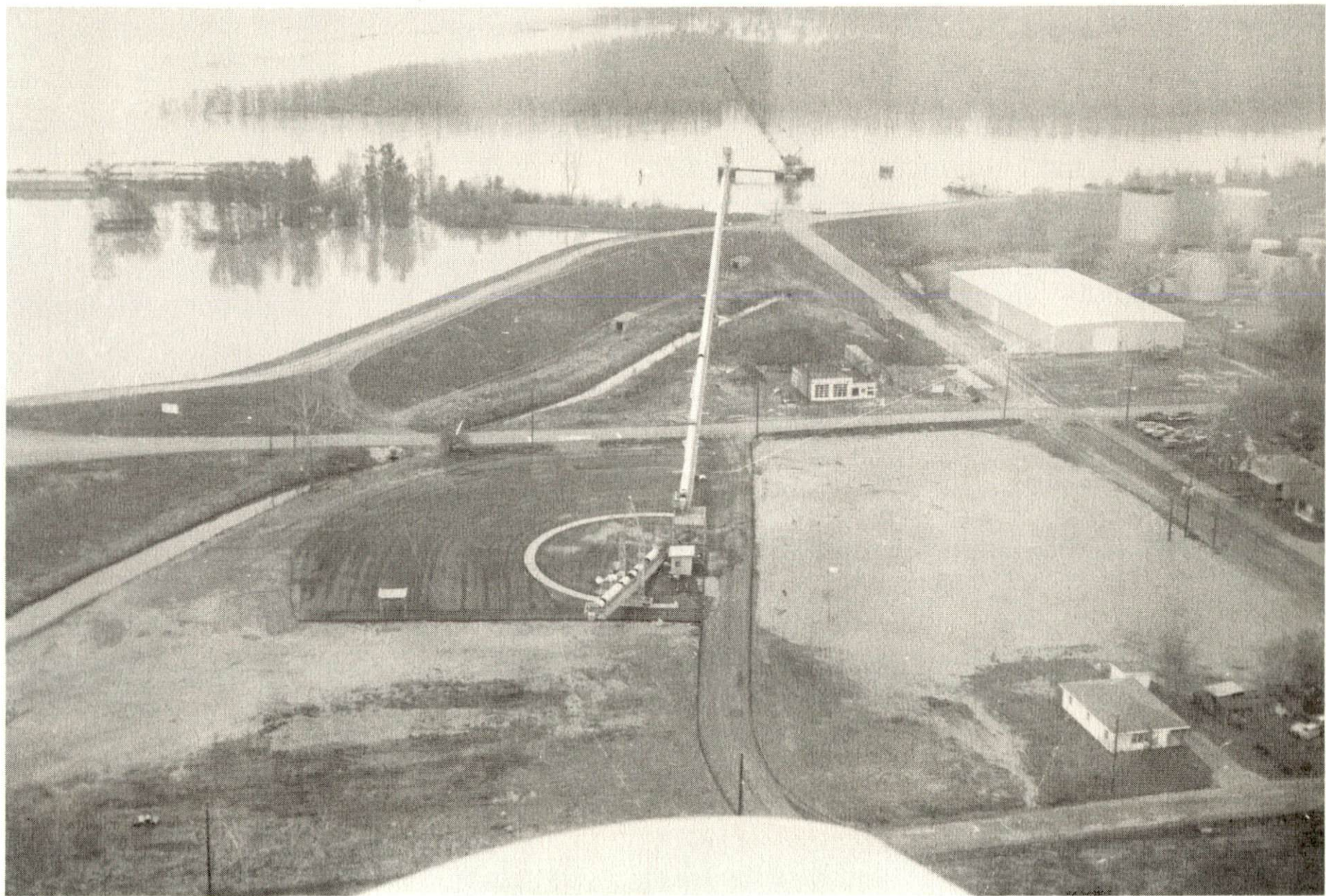
AERIAL VIEW OF HICKMAN-FULTON COUNTY RIVERPORT
