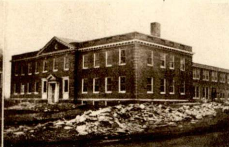
Dairy Products Building.
