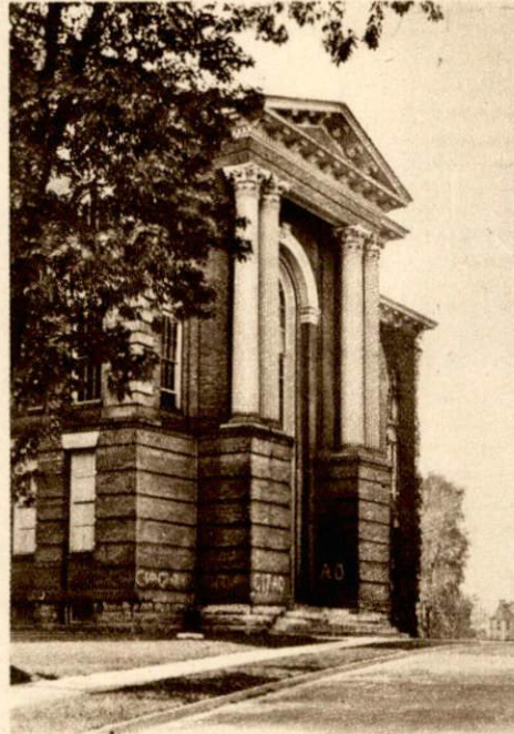
Main Building, Centre College, Danville, Ky.
