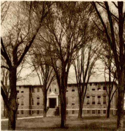
THE ADMINISTRATION BUILDING One of the five on the campus
