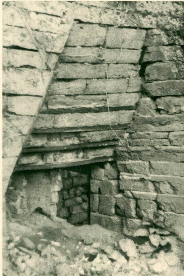
Remains of old furnace on Slate Run, where cannon balls were made and shipped to New Orleans during the War of 1812
