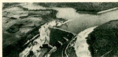
Dix Dam, Harrodsburg, Ky. Largest rock-filled dam in the world.
