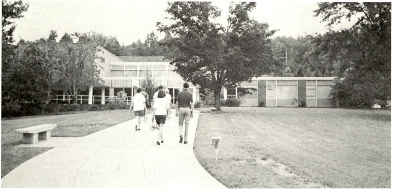
Cumberland Gap National Historical Park Visitors Center Museum and Administration Building
