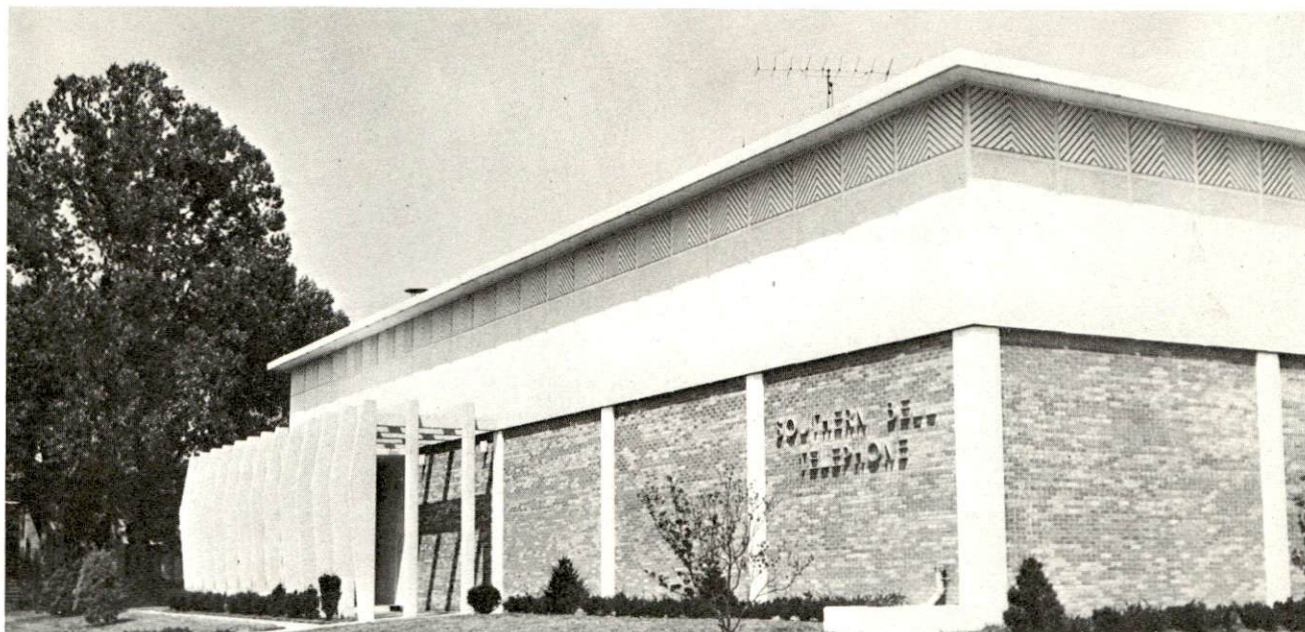
Southern Bell Telephone and Telegraph Co.
